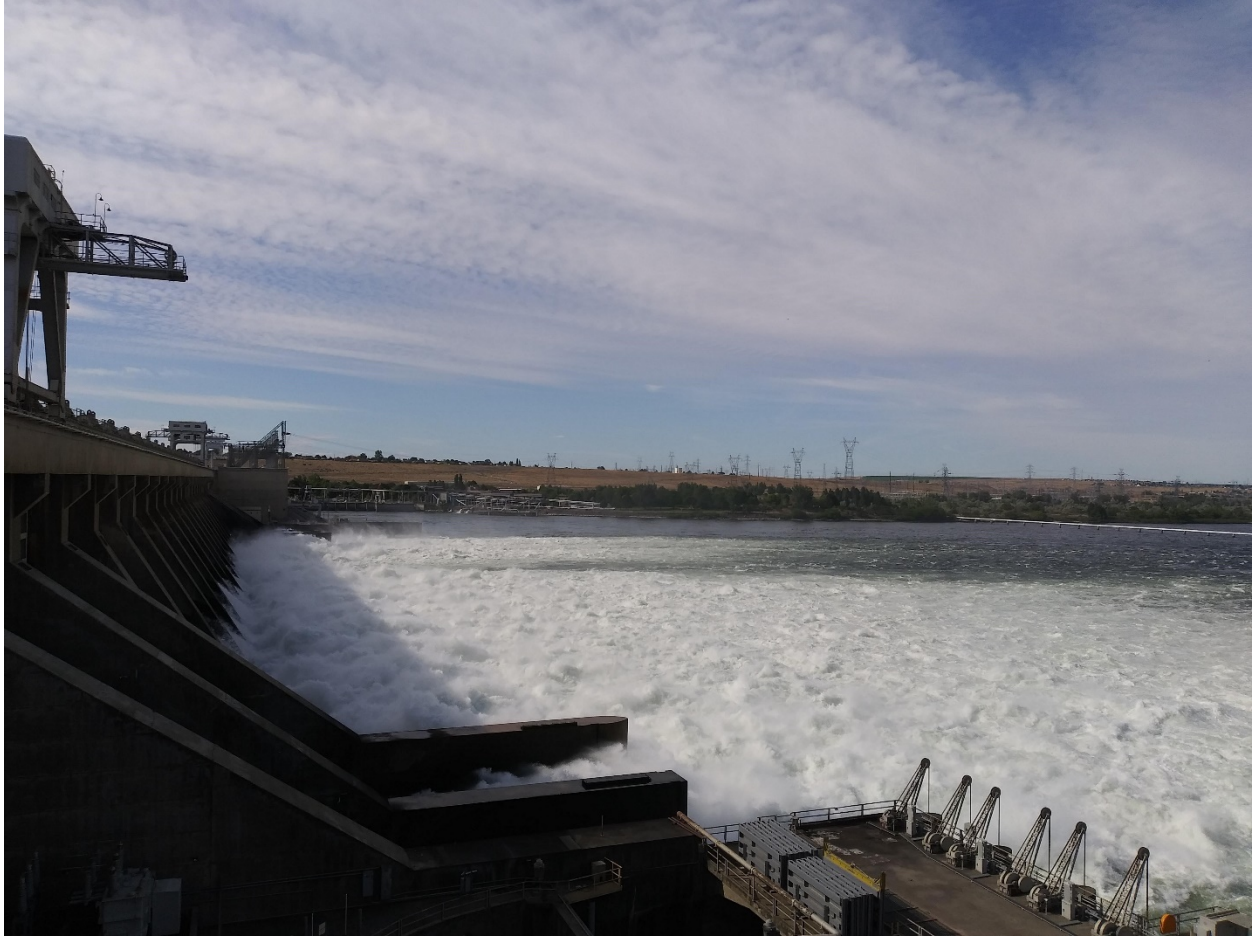
Spill pattern bay 15 closed.
