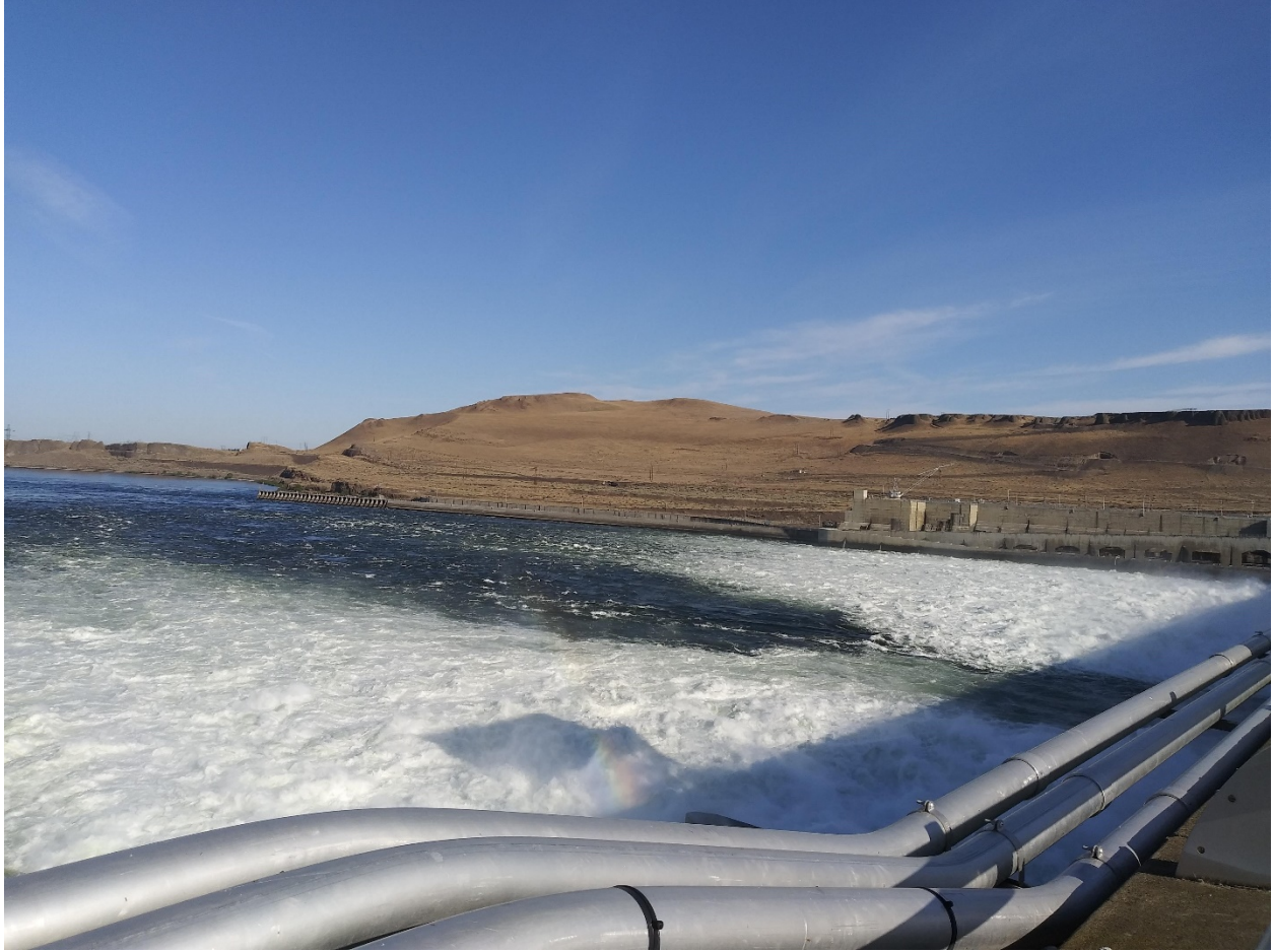
Spill pattern when removing hoist parts.
