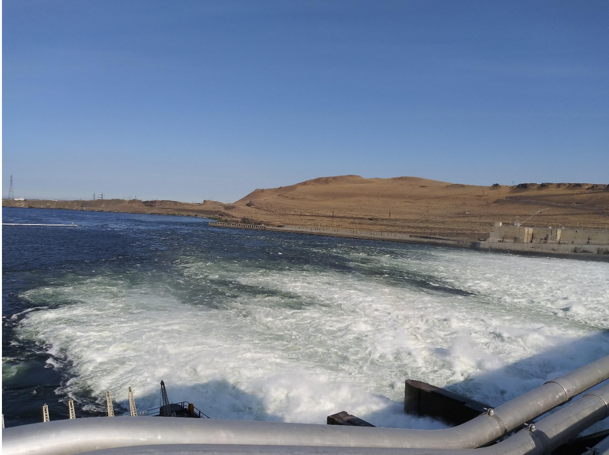
Spill pattern with bays 15 and 20 closed.
